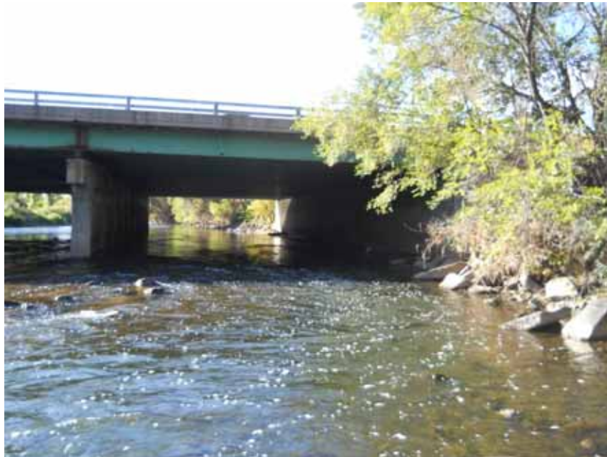
Photo 1 — South Platte River looking south toward the existing US 6 bridge
