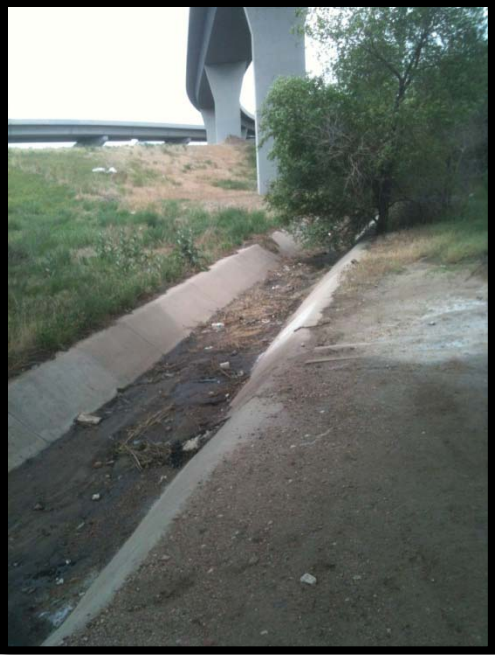
Photo 11 — Concrete lined ditch north and east of US 6 and I-25
