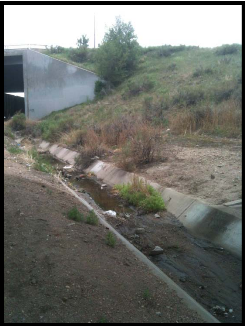
Photo 12 — Concrete lined ditch north and east of US 6 and I-25
